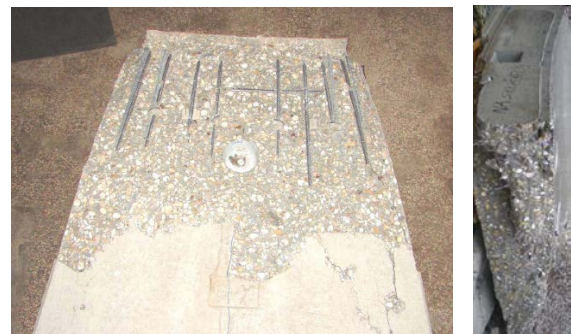
Figure 10. Comparison of damaged key segments after reaching their capacity:
