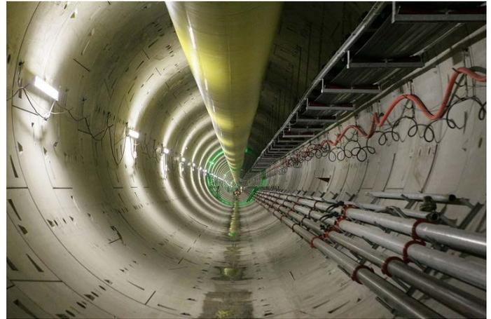
Figure 13. Segmental lining of a running tunnel on the Line A of Prague metro
