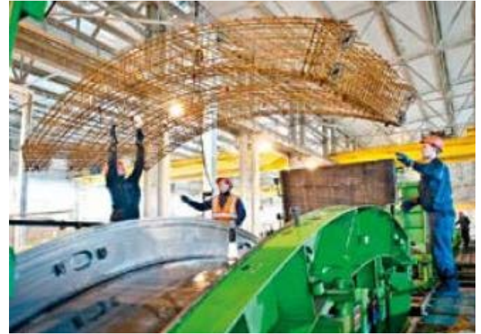
Figure 7. Steel reinforcement cages placed to moulds during production of steel bar reinforced concrete segments
