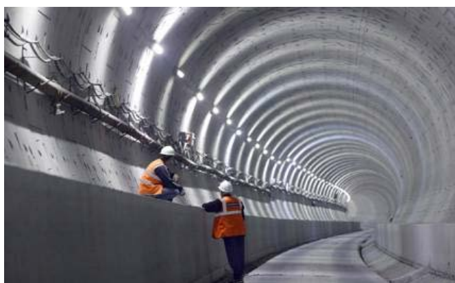
Figure 10. Tunnel CTRL with SFRC segments
