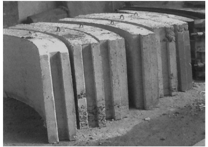
Figure 8. SFRC segments generated and tested in the Czechoslovakia in 1984 - 1988
