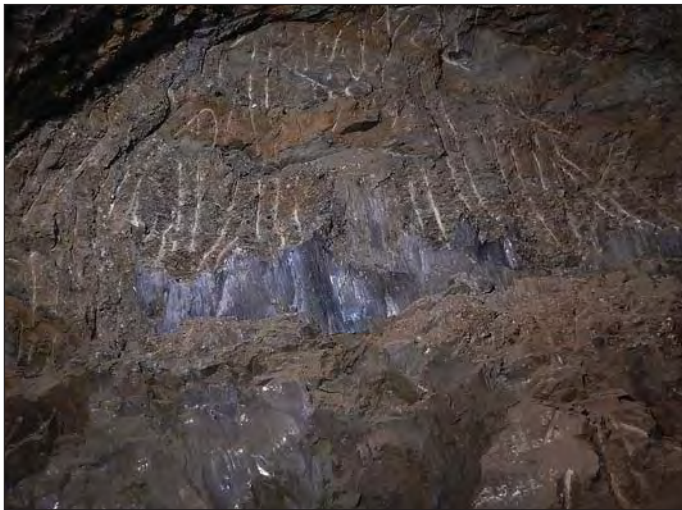
Obr. 5 Detail vyhlazené plochy v tunelu DG1 TM 1419 Fig. 5 A detail of a slickensided surface in the DG1 TM 1419 tunnel
