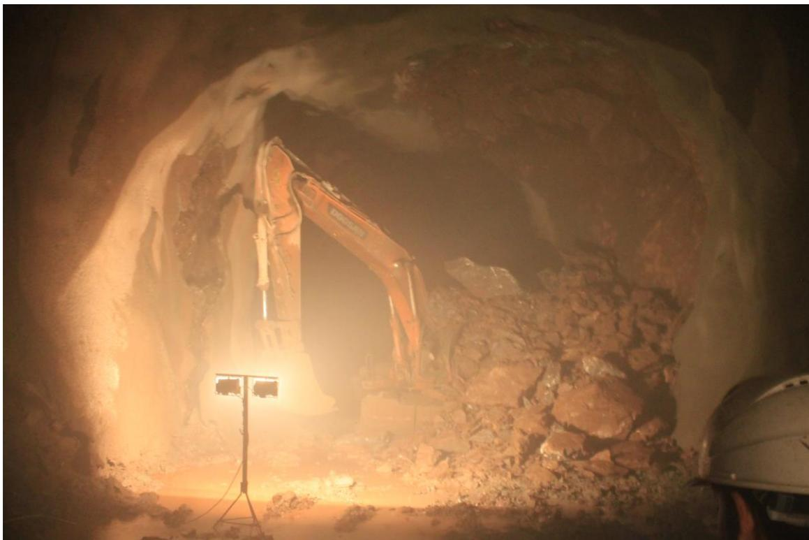
**Figure 4.** An excavator buried by collapsed rock support and surrounded rock mass. The photo taken during time when rock was still falling and shotcrete lining was cracking. An excavator operator was pulled out alive.
