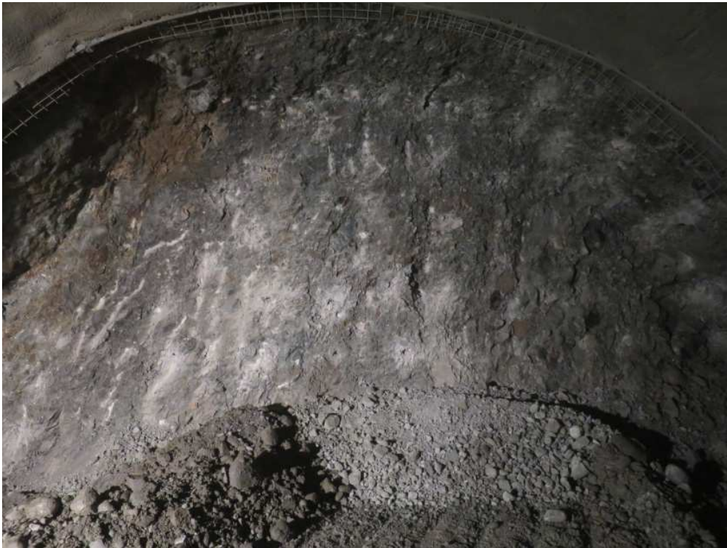
Figure 3: Tunnel face with exotic conglomerates
