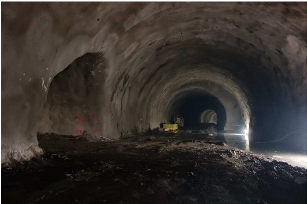
Figure 4: Primary tunnel lining of an emergency bay with a cross-passage in the STT
