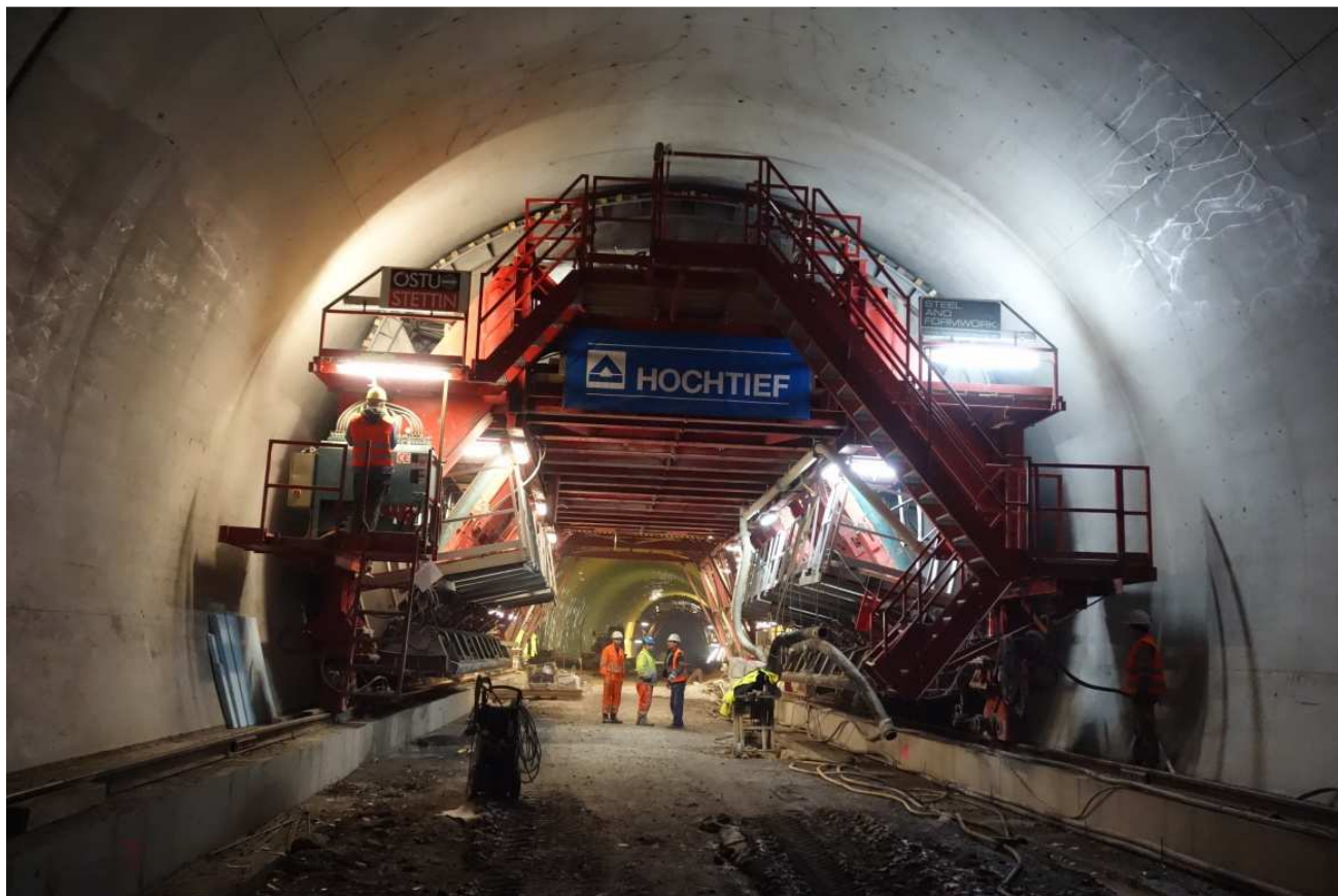
Figure 7: Works on the final tunnel lining
