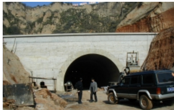
PORTAL - TUNNEL CHEN JIA SHAN
