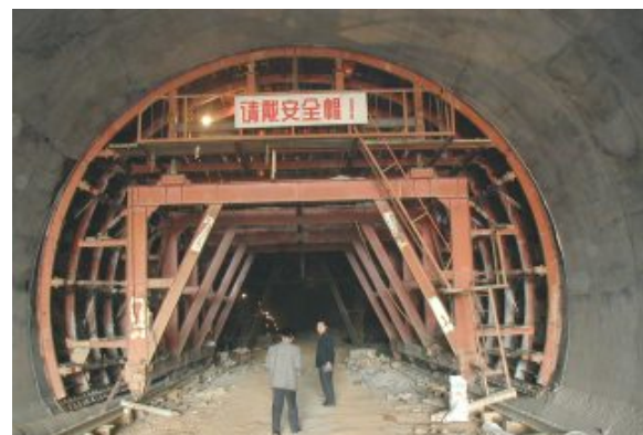
SCAFFOLDING OF TUNNEL CHEN JIA SHAN
