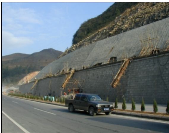
ROAD OPENED- FINISHING WORKS
