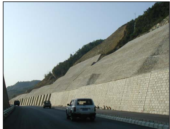
LARGE RETAINING STRUCTURES PROTECT THE ROAD
