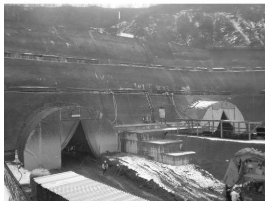
Figure 3. View of surcharging concrete block between tunnels
