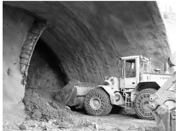
Figure 2. Excavation with splitted top heading
