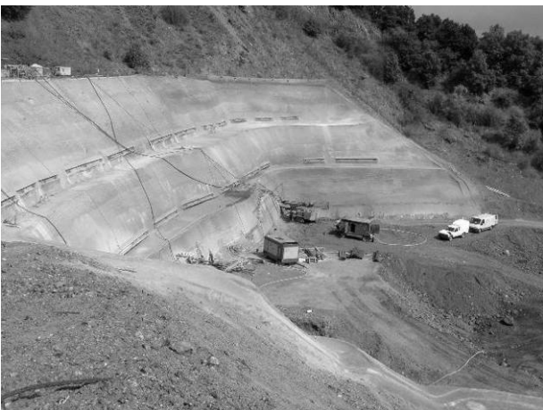
Figure 1. Prague's portal area prior start of excavation
