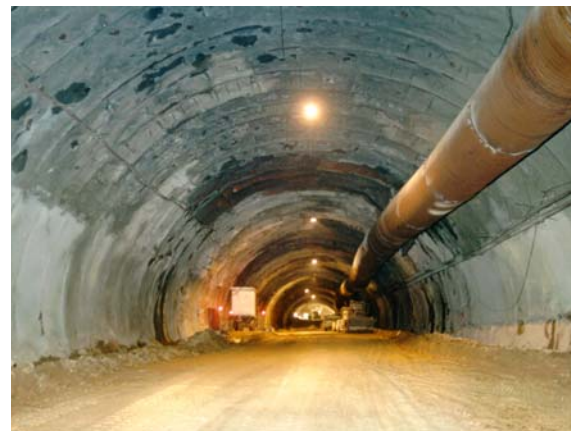
EXCAVATION TO FULL PROFILE
