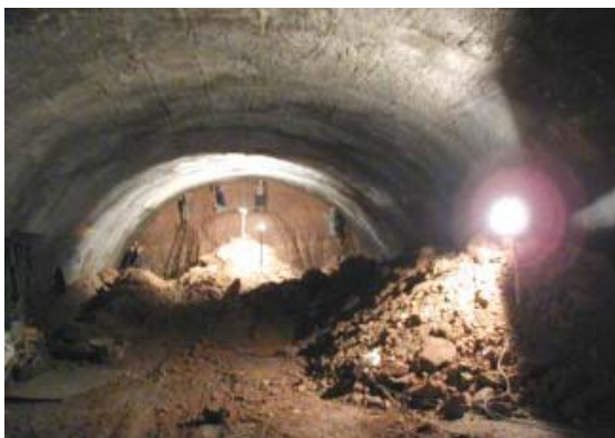
KALOTA - TUNEL CHENG WANGZHUANG
